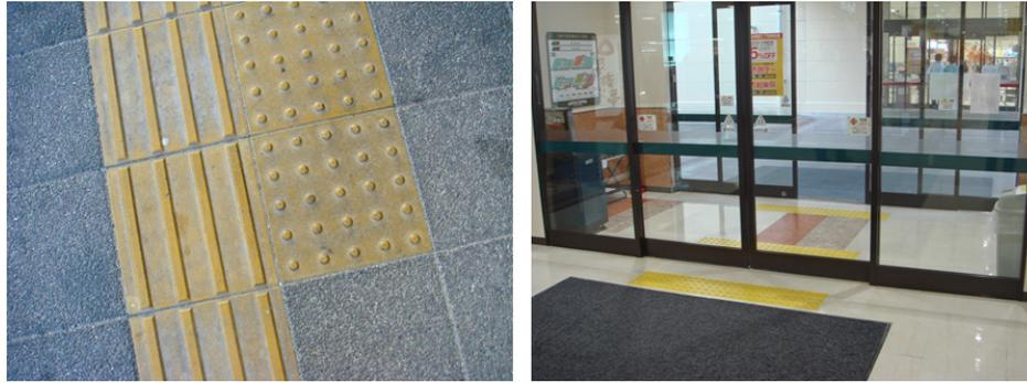
Figure 7.10: Detectable warning surfaces for visually-impaired pedestrians are common in public spaces in Japan. Some robots cannot safely traverse these surfaces.
