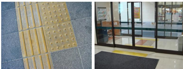
Figure 10. Detectable warning surfaces for visually-impaired pedestrians are common in public spaces in Japan. Some robots cannot safely traverse these surfaces.
